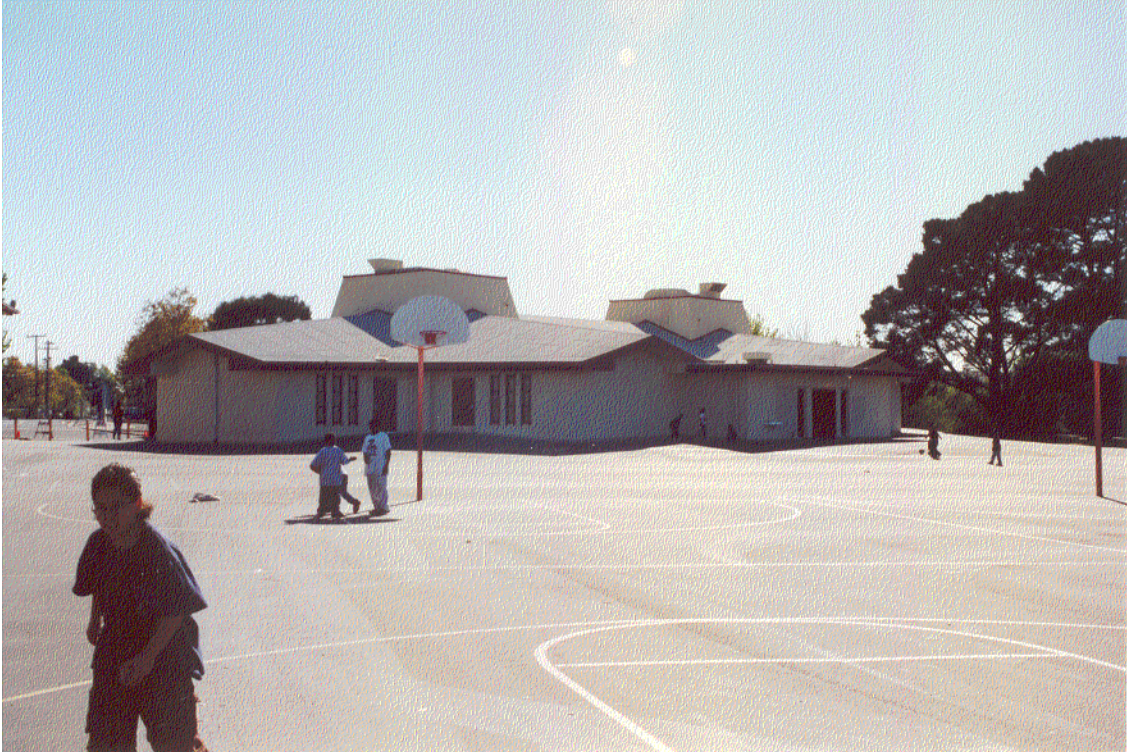
Figure 11: Unit A (classroom building) north face
