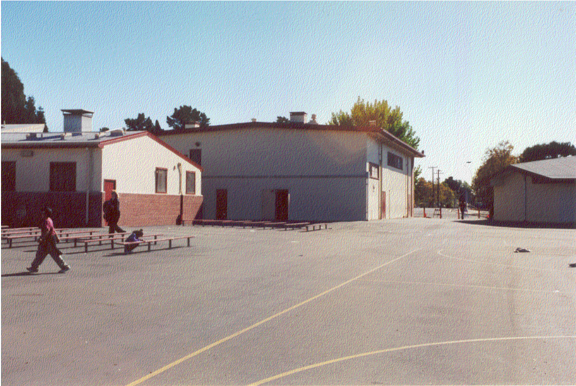
Figure 10: Unit B (multipurpose building) north face
