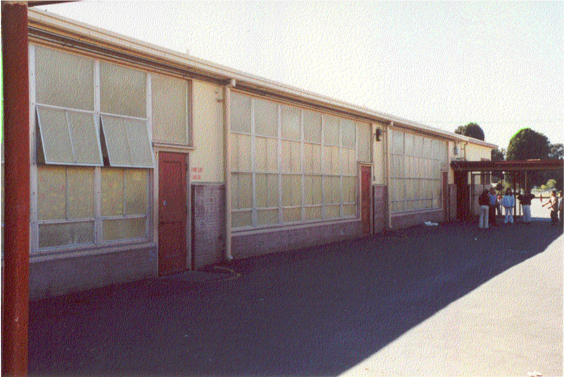
Figure 4: Unit D (classroom buildings) north face
