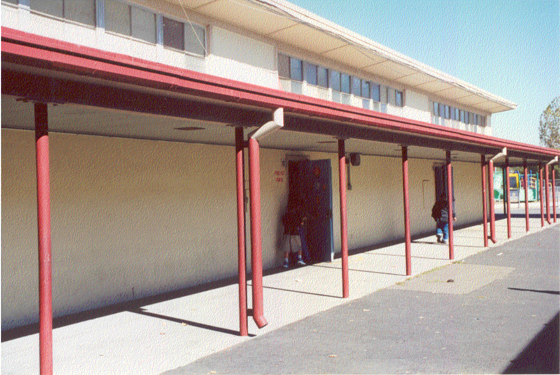
Figure 5: Unit C (classroom building) south face
