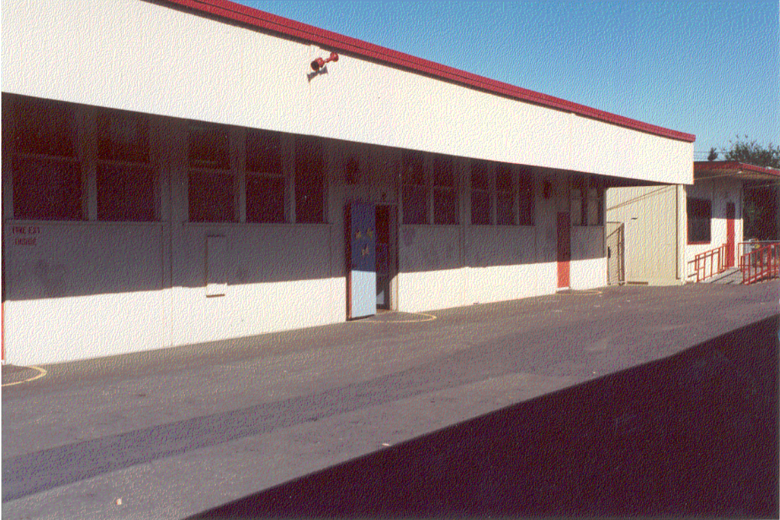
Figure 7: Unit E (classroom building) south face
