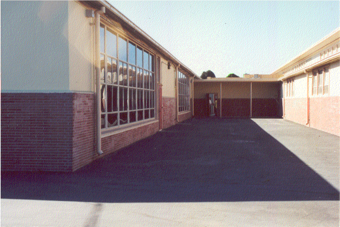
Figure 3: Unit D (classroom buildings) east face
